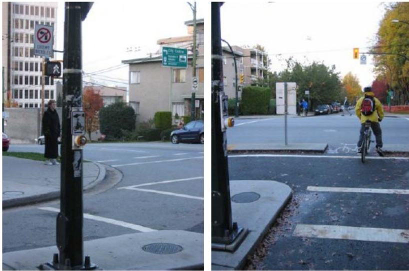
Figure 24: Example of a bike box with cyclist controlled signals
